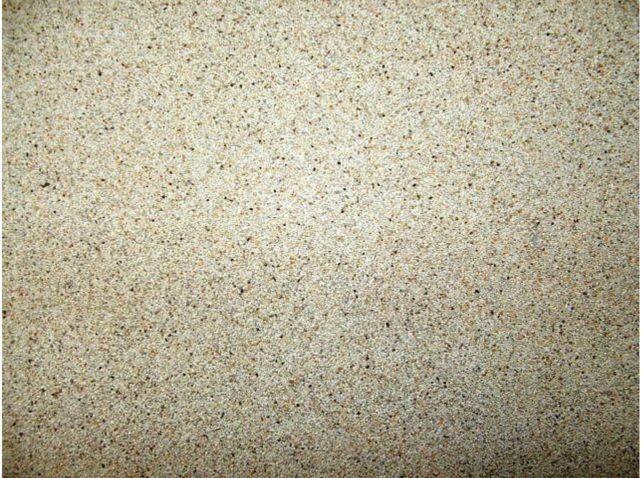
Photograph No.1 Top surface of sheet membrane
